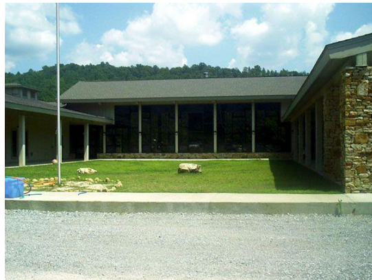
Entrance from the parking lot
