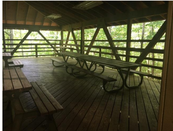
Deck attached to main building.
